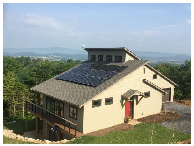
7.2 KW solar array includes 24 300-watt, 60-cell Canadian Solar monocrystalline modules. A SolarEdge inverter (located in lower ground floor) with DC optimizers completes the system.
